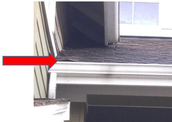
There are a number of problems with gutters and downspouts that require repair as they are spilling water onto siding and trim and causing decay
